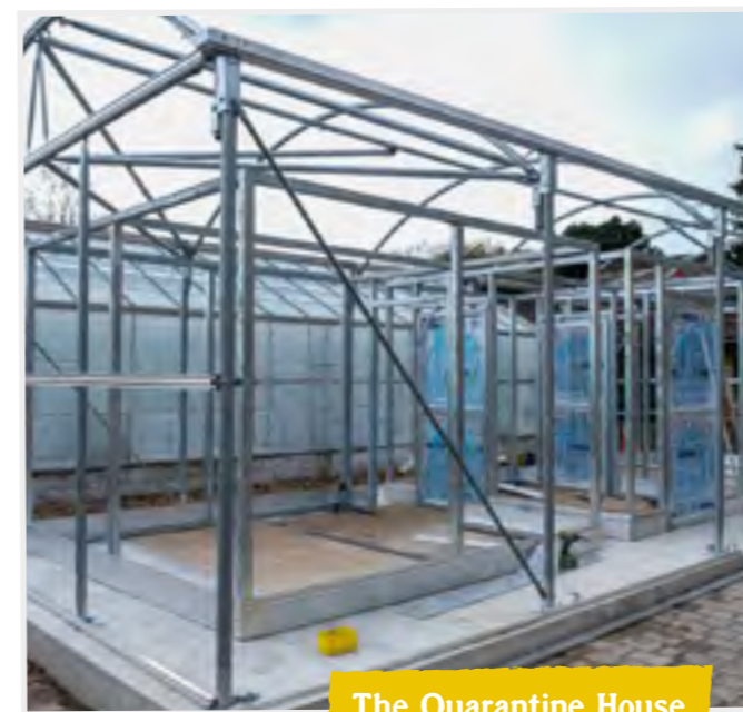
The Quarantine House during construction
